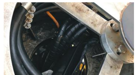
Technician Terminating Cables
